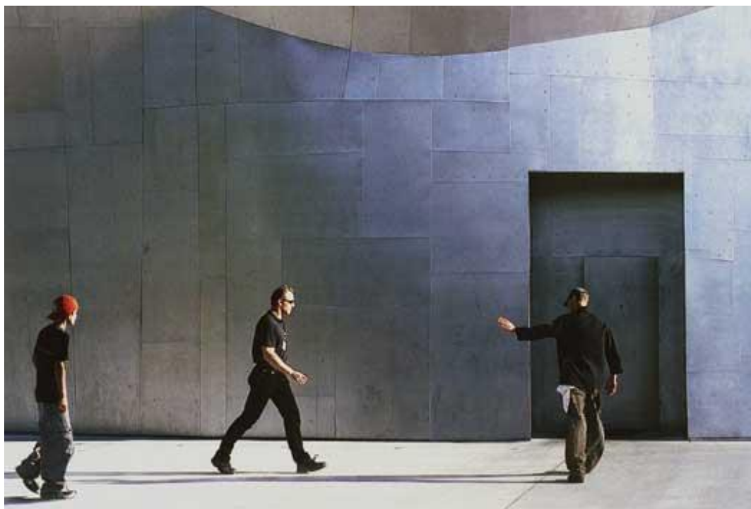
Figure 21: Metal walls in room with colored Break-Out Blocks. Panels riveted together in a disorderly, yet functional pattern
